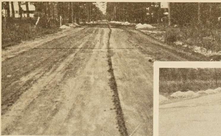
BELOW: SAND-CLAY BASE PRIMED AND READY FOR THE STONE TO BE SPREAD.]
